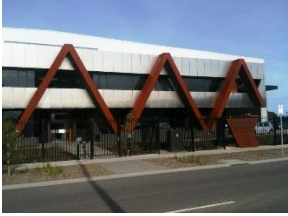
The standard of architecture at Logis is exceptionally high for an industrial estate. [Source: Nathan Alexander]
