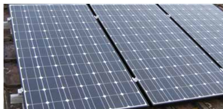
Tilted roof-mounted solar panels.
