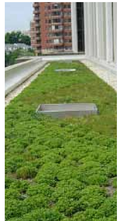
Example of a low-irrigation green roof.
